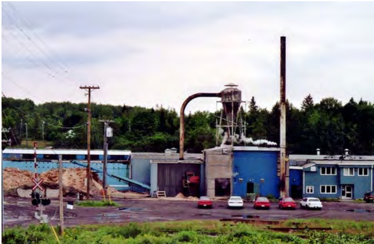
Photo 6.2.9 Atcon veneer mill, Napadogan, New Brunswick (Janice Cook, July 25, 2006). Located on Route 107 between Williamsburg and Juniper, the mill produced veneers for furniture, flooring, doors, skateboards, and musical instrument cases. P194-598 Miscellaneous photographs collection, Provincial Archives of New Brunswick (PANB n.d.).
