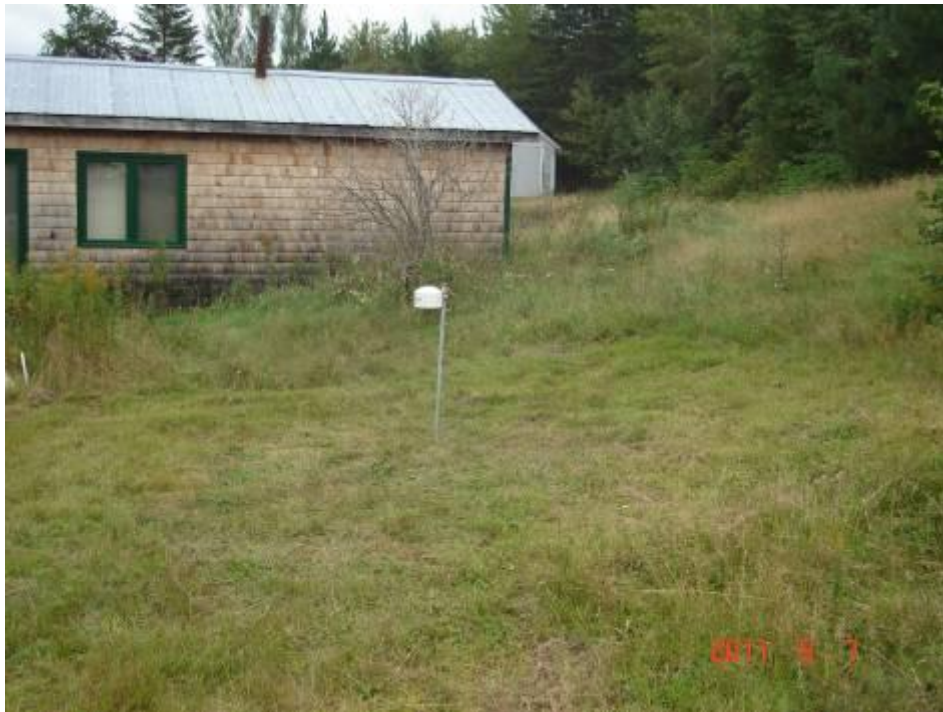
Figure 3.3 Passive Samplers Monitoring Location – 29 Second Street, Napadogan, NB
